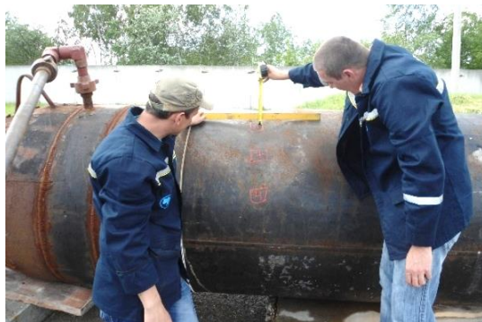
Figure 6. Monitoring of the dentdepth during the reservoir test
