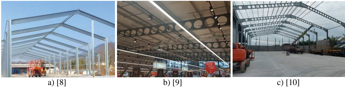
Figure 1. Elements of pitched roof systems formed by solid-web (a), single-pitched (b) and double-pitched (c) perforated steel beams.
